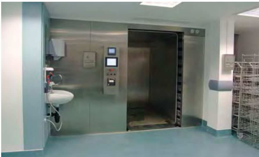
Autoclaves are often used in hospitals, to sterilize surgical instruments.
